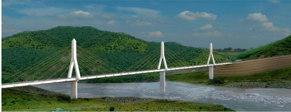
Figure 1. General view of the bridge
